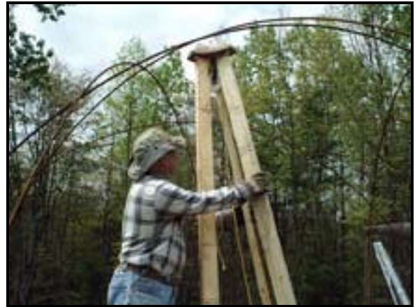
Figure 28 - Remove the 53" Spacers, rope and pulley and take the tripod down.
