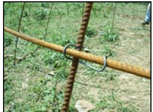
Figure 30 - Use Rebar Clip to fasten at 33" height
