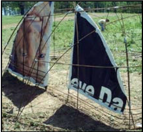
Figure 49 – Cover the inside wall first
