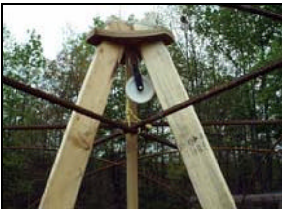
Figure 25 - Dome in Up Position
