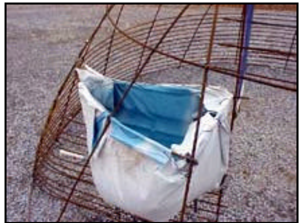
Figure 39 - You are now creating a frame for a vinyl water reservoir
