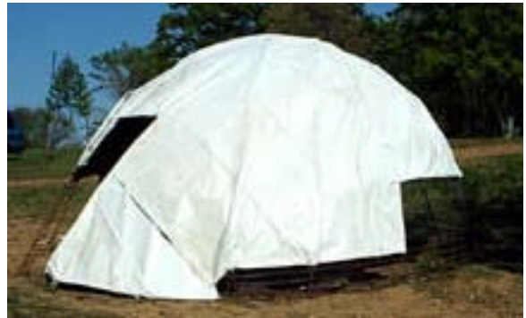
Figure 52 - The fabric wraps around the doorframe and creates a fabric door to cover the grain.
