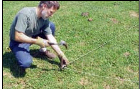
Figure 10 - 3 Layout cables locate ground stakes
