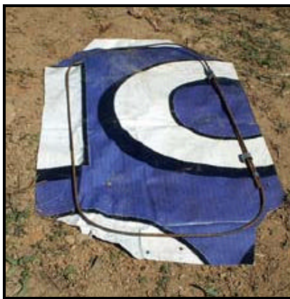
Figure 53 - Create the door by bending a rectangle 26" X 48". Preinstall two 1 1/2" Galvanized rings to use as door hinges. They will attach to a door jam placed inside the inside wall.
