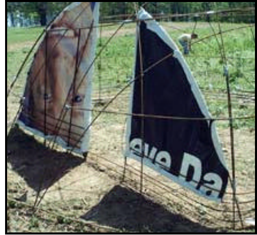
Figure 37 - You have just created the frame for the inside walls
