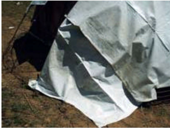
Figure 51 - Place a piece of fabric over the feed storage area and rivet it in place.
